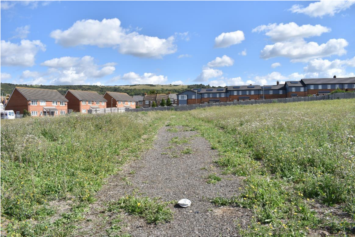
Plate 16: View along the access road internally within the PDA (Facing NE).
